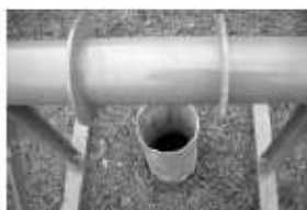
Roller must be aligned with the casing.
